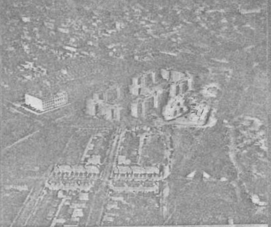
IX. A Birdseye View of Boulevard Gardens Project Under Construction
