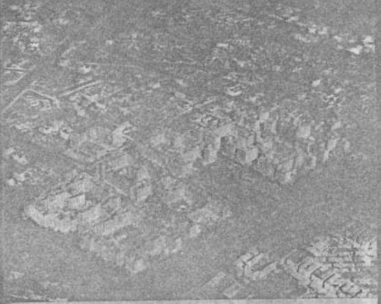
VIII. Birdseye View of Hillside Housing Corporation Under Construction
